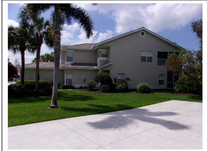
ROOF GEOMETRY – Gable / Other Roof Shape
