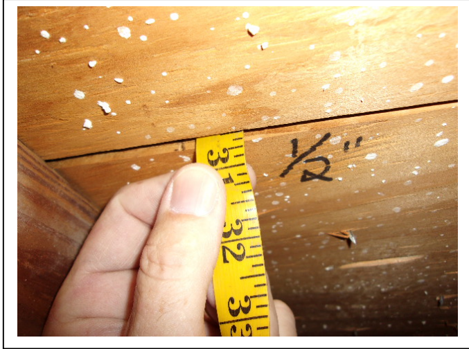
ROOF DECK THICKNESS – 15/32 to 1/2 inch plywood
